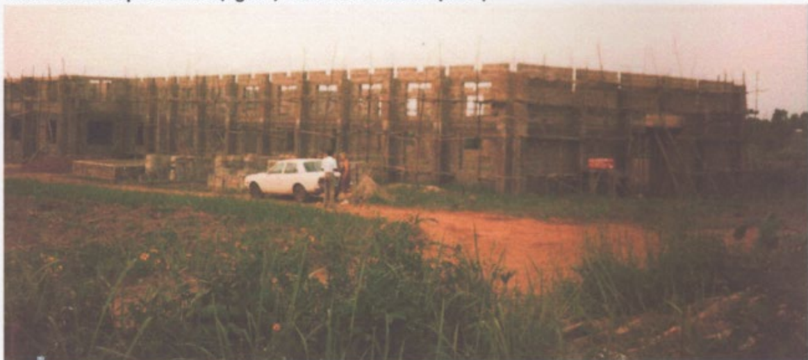
The Ikogosi Baptist Church, under construction (1972)
